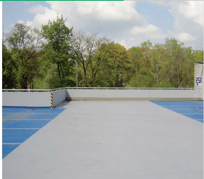
▲ Grade-level parking lotb Zlin
